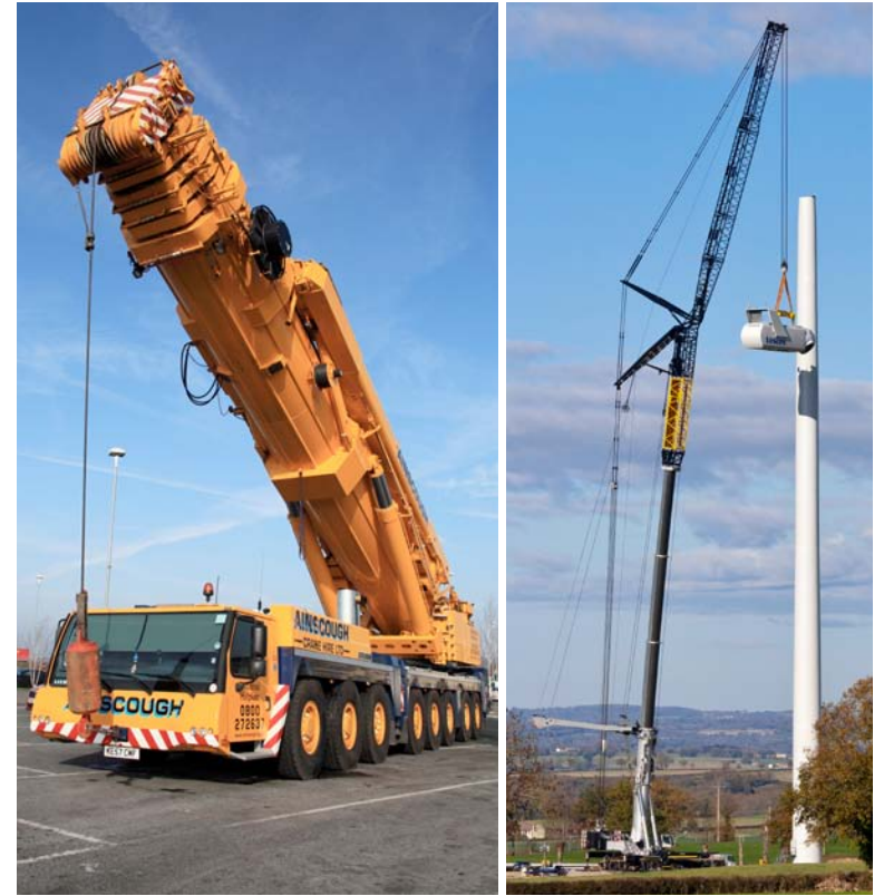
Heavy cranes are big enough to set up structures.
